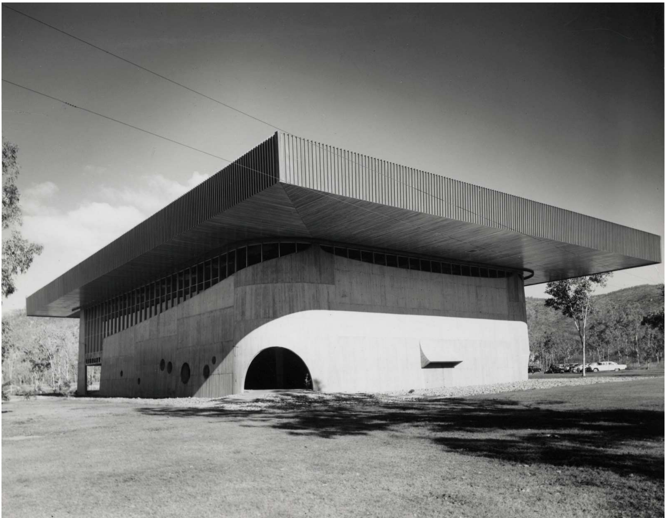
University College of Townsville Library in Townsville, Queensland [now known as Eddie Koiki Mabo Library at James Cook University, built in 1968], c.1968. Photograph by Beverly Studio. Image no. 6523-0001-0413
