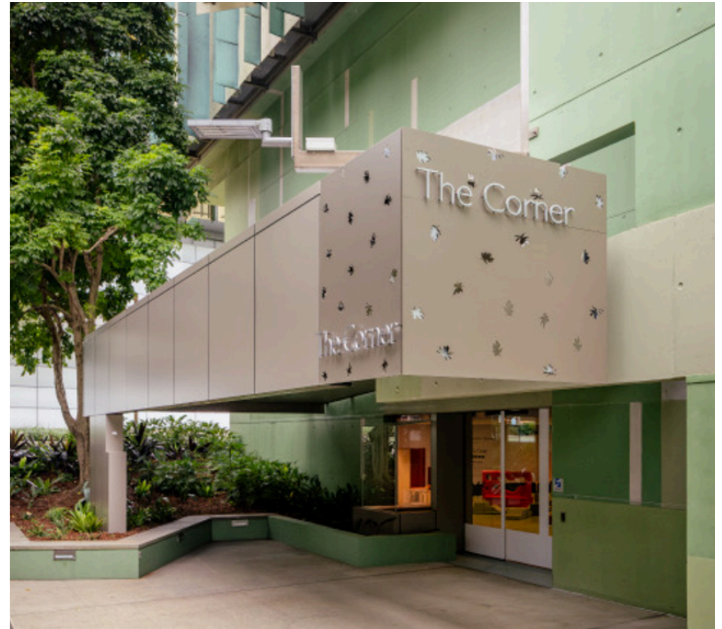
Big metal canopy above the doors into The Corner.
